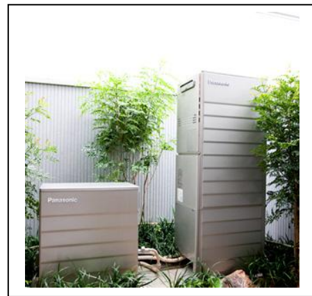
Figure 5: Fuel cell in a residential house
